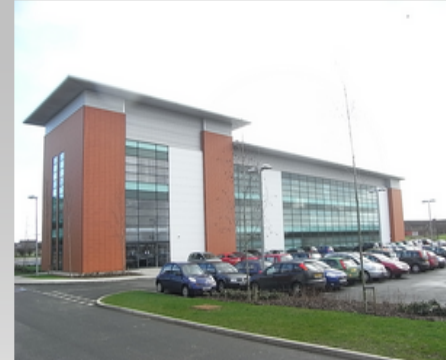
Q16 Building, Quorum Business Park, Newcastle
